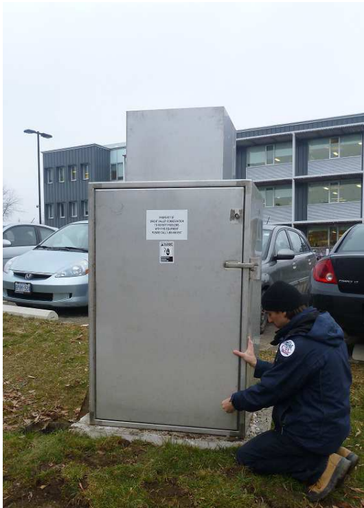
Installation of exterior housing for performance assessment equipment
