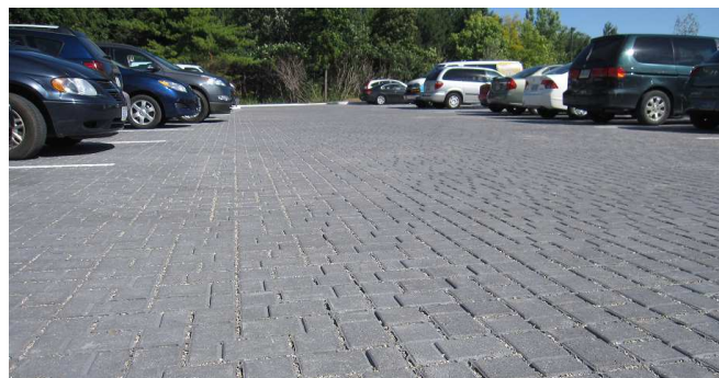
Photograph of the expanded parking lot after construction
