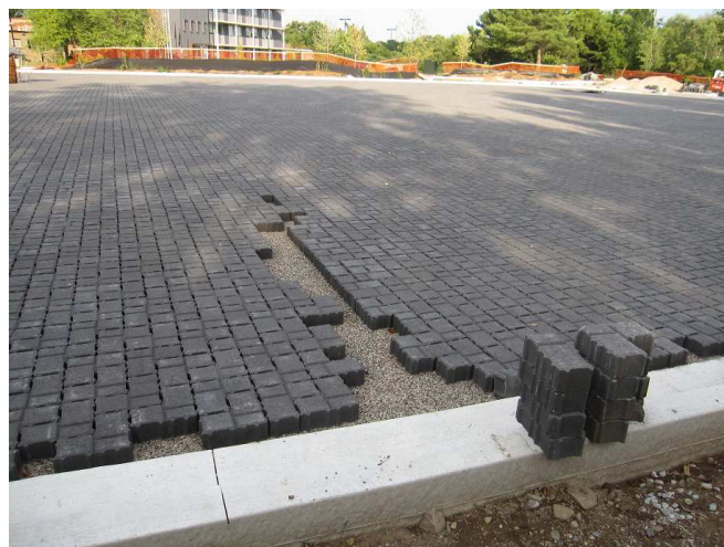
Permeable pavement expansion. Parking lot during construction
