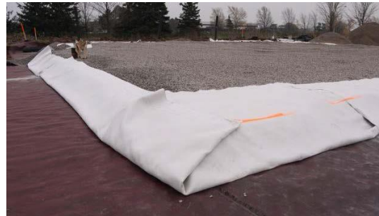
Figure 7: Geosynthetic clay liner and \frac{3}{4} inch clear stone aggregate
