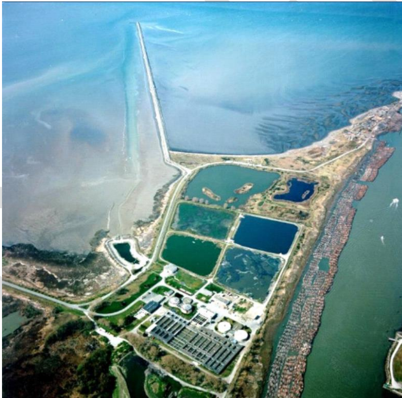
Figure A-2. Iona Island WWTP (Photo courtesy of Metro Vancouver)
