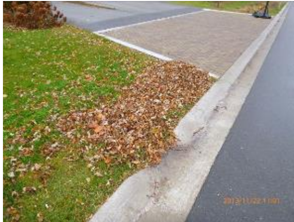
Figure 5-3 Leaves blocking the inlet and partially covering the bioswale, which could impede flow and reduce performance
