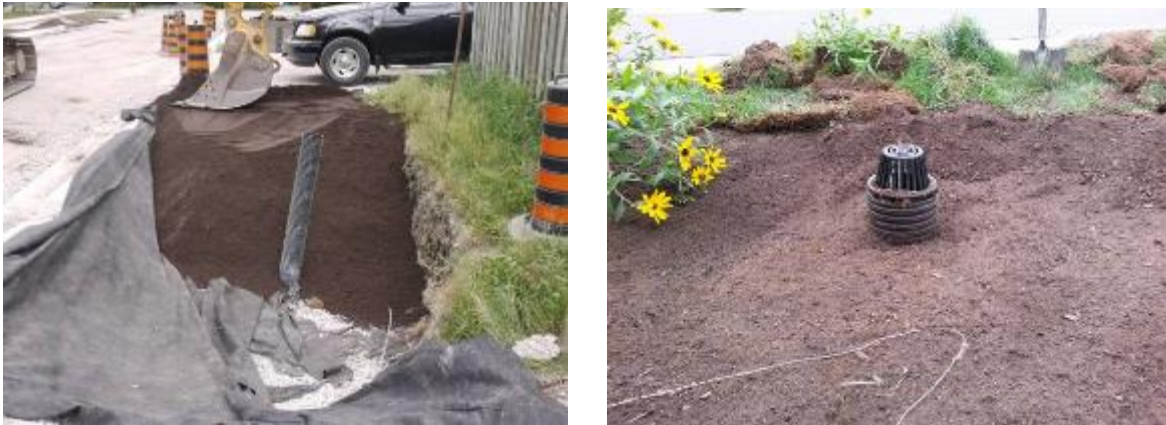
Figure 3-6 Overflow pipe with debris screen (left), Soil media being installed around an overflow pipe (right)
