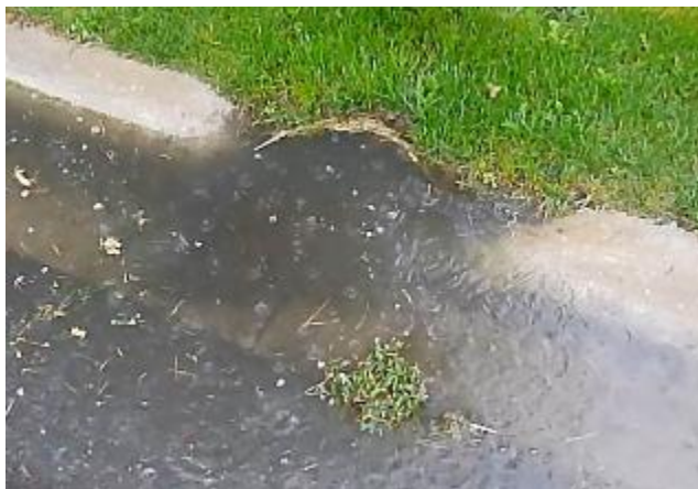
Figure 5-6: Inlet with incorrect grading, water is unable to enter the bioswale
