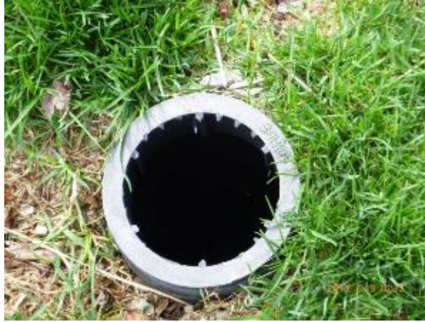
Figure 5-4 Missing overflow cap at the outlet pipe in the Spring after the snow has melted
