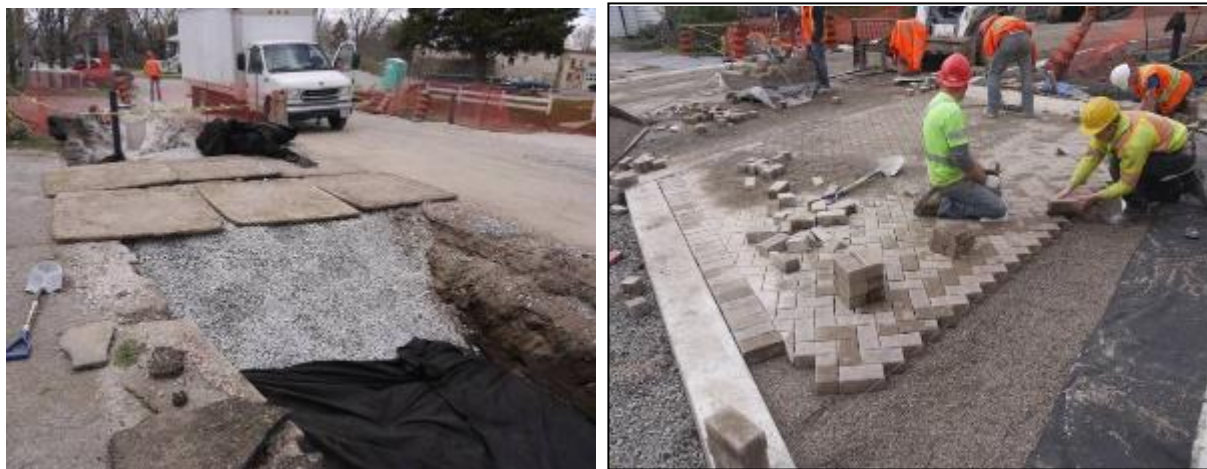
Figure 3-3 Preparation of permeable pavement driveway base materials (left) and permeable pavers (right)
