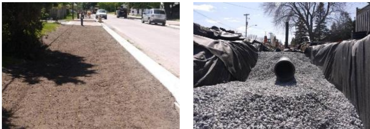
Figure 3-5 Bioswale with underdrain in gravel layer (left), Engineered soil mix within the bioswale (right)
