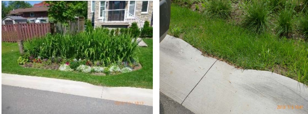
Figure 3-4 Curb cuts allow road runoff to enter the vegetated bioswales
