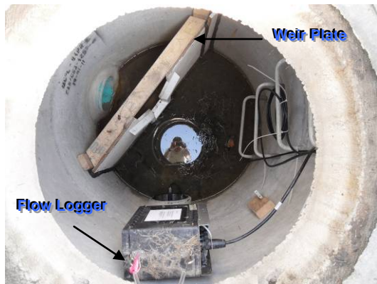
Figure 2-1: Flow Logger and Compound Weir
