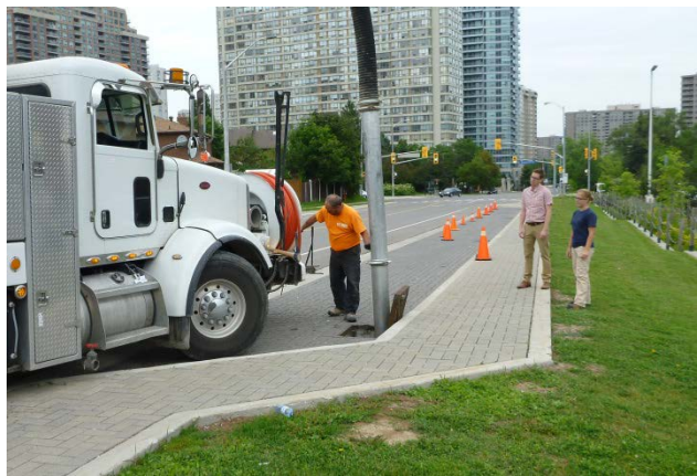
Figure 4-20 Catch basin maintenance in July 2015
