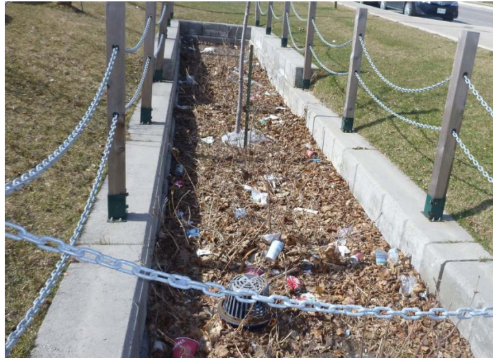
Figure 4-19 Debris and leaf litter in a bioretention cell
