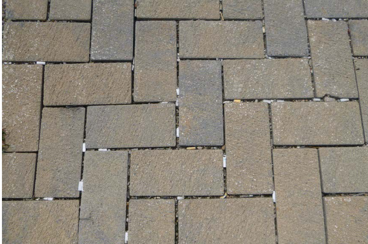
Figure 4-21 Cigarette butts caught in permeable paver joints
