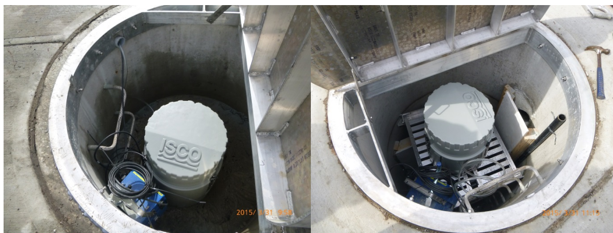
Figure 4-1: Monitoring equipment installed in inlet chamber (left) and outlet chamber (right)
