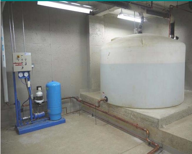
Indoor rainwater storage tank, located in the basement
