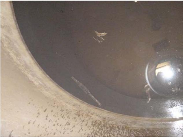
Accumulated sediment and debris in the rain tank.
