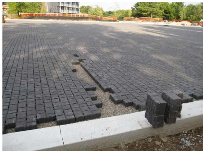
Permeable pavement expansion parking lot during construction
