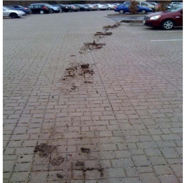
Picture showing mud tracking from construction vehicles
