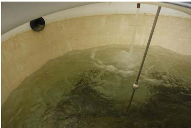
Interior view of rainwater storage tank during top-up filling process
