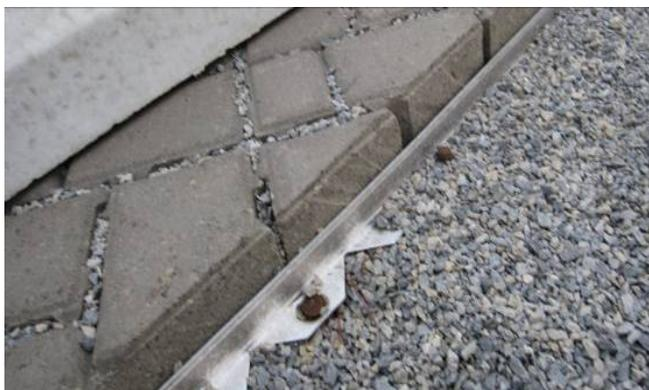
Close-up photograph of permeable paver edging restraint
