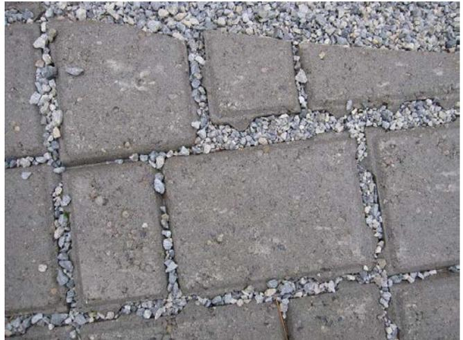
**Close-up view of the chip stone used in-between pavers**
