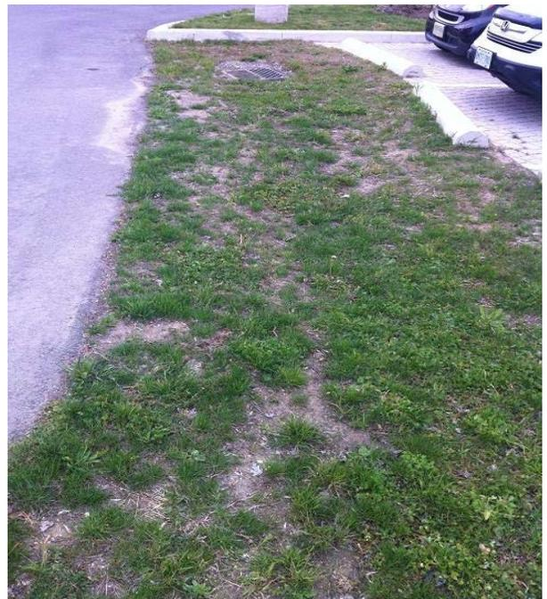
Grass swales, with erosion channels (rills)
