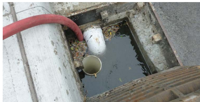
Figure 8: Water test in the east catch basin
