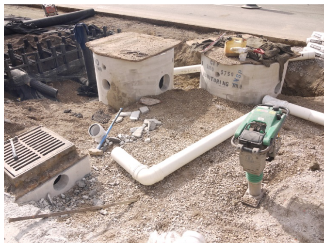
Figure 7: Installation of monitoring chambers and pipe connection
