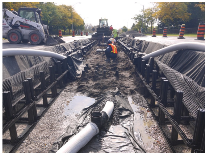
Figure 5: Distribution pipe installation and bioretention media inspection
