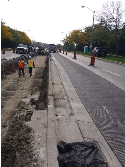
Figure 13: Catch basin protected with erosion and sediment control
