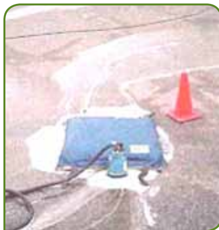
Cover storm drain inlets to prevent wash water from entering storm drain.
