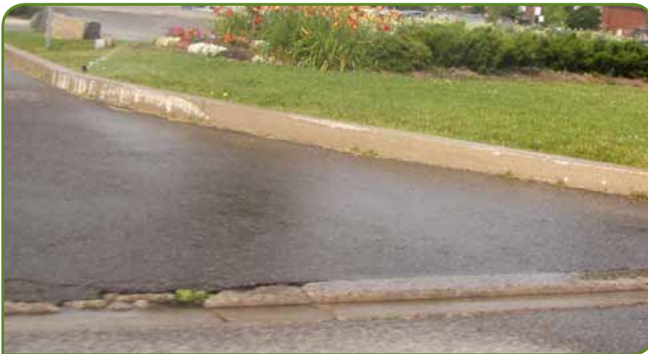
Non target Irrigation sprinklers are also watering the pavement.
