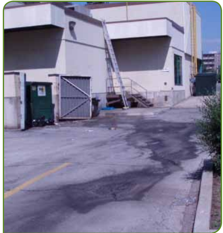
Evidence of waste moving towards the storm sewer.
