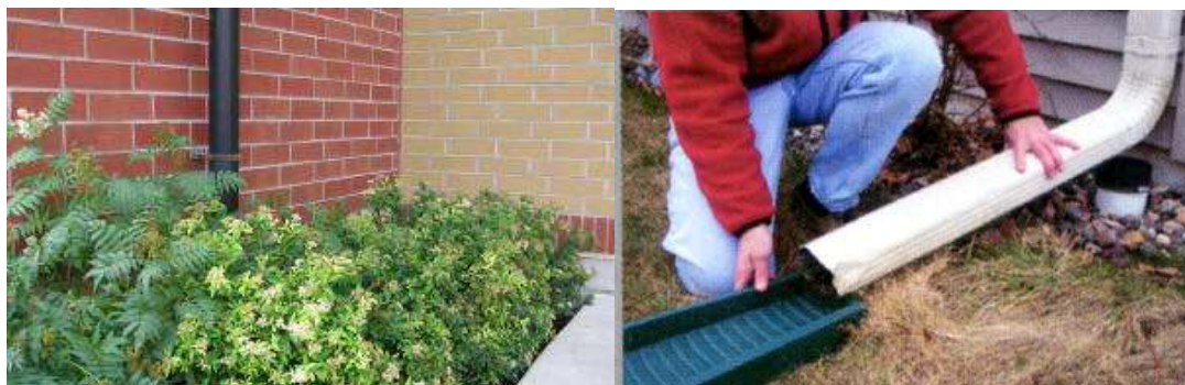
Figure 3.28 External roof leaders draining to lawns in the watershed
