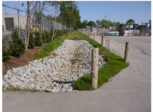
Sediment trap on the west side of the property
