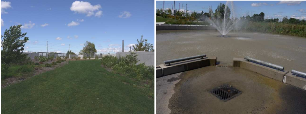
Figure 3.3 Green Roof over washroom building (left) and receiving pond area retaining water used for irrigation (right) at Lakeside Park in the City of Mississauga.
