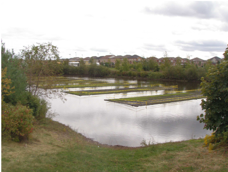
Figure 3.26 8,000 ft 2 of Floating Island Installed at Pond 10 in Northwest Brampton
