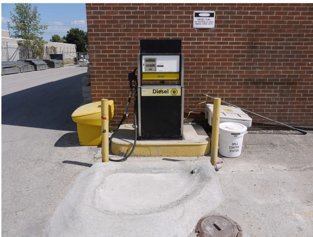
Spill containment sump installed
