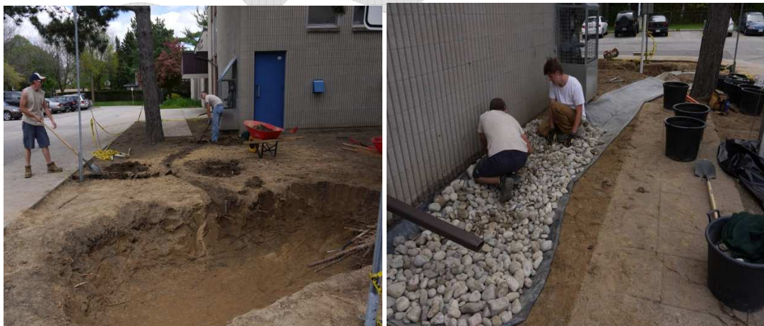
Figure 3.10 Construction of the rain garden at Green Glades Public School
