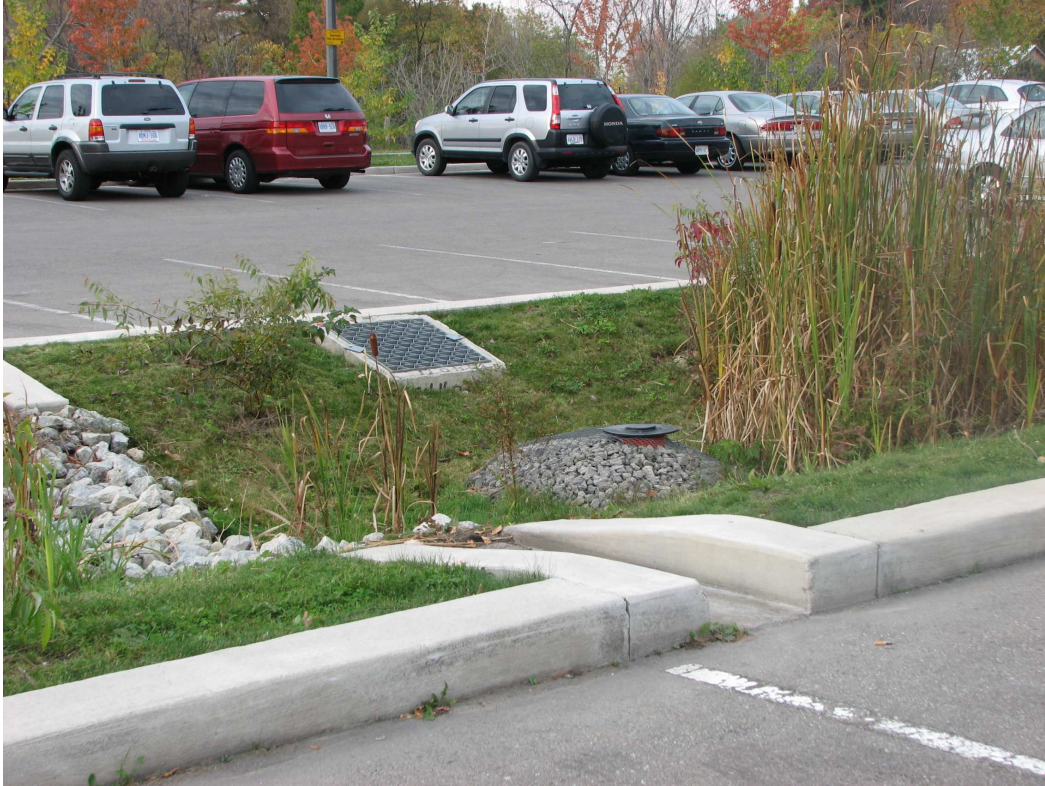
Figure 2.32 Example of an island landscaping retrofit at Riverwood Conservancy, in Mississauga. This can be applied to apartment buildings
