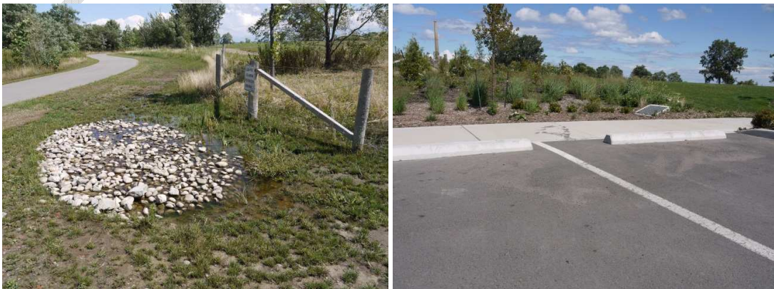
Figure 3.2 Swale draining off-leash dog park (left) and bioretention cell receiving runoff from parking lot (right) at Lakeside Park in the City of Mississauga.
