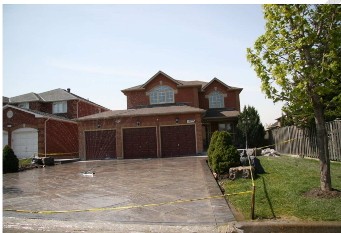
Figure 2.19 Example of driveway washing, non-target irrigation
