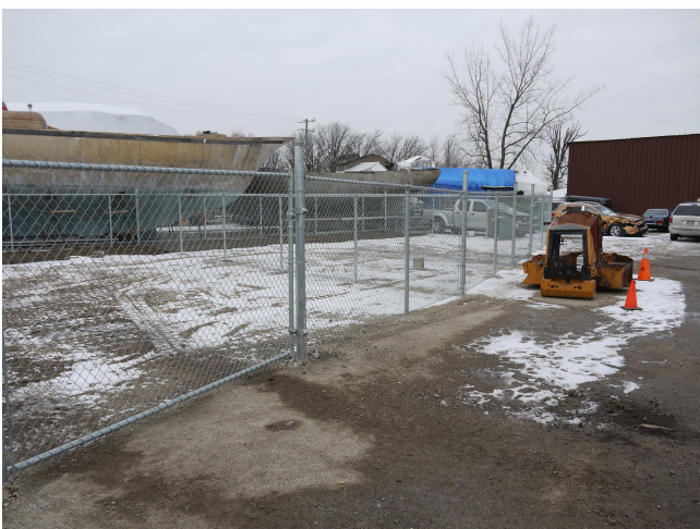
New fencing installed
