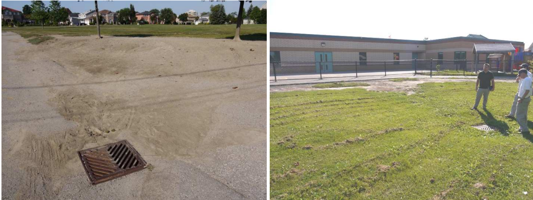
Figure 3.7 Examples of unsustainable drainage features at Cherry Tree public school: sediment draining to catch basin, mowed grass draining to catch basin
