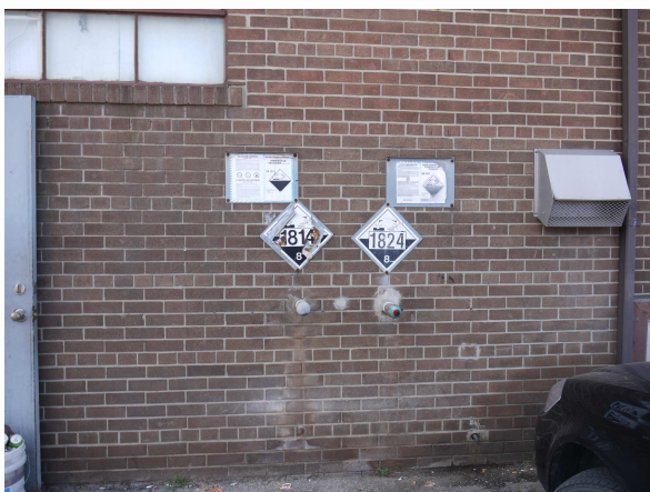
Filling lines before construction
