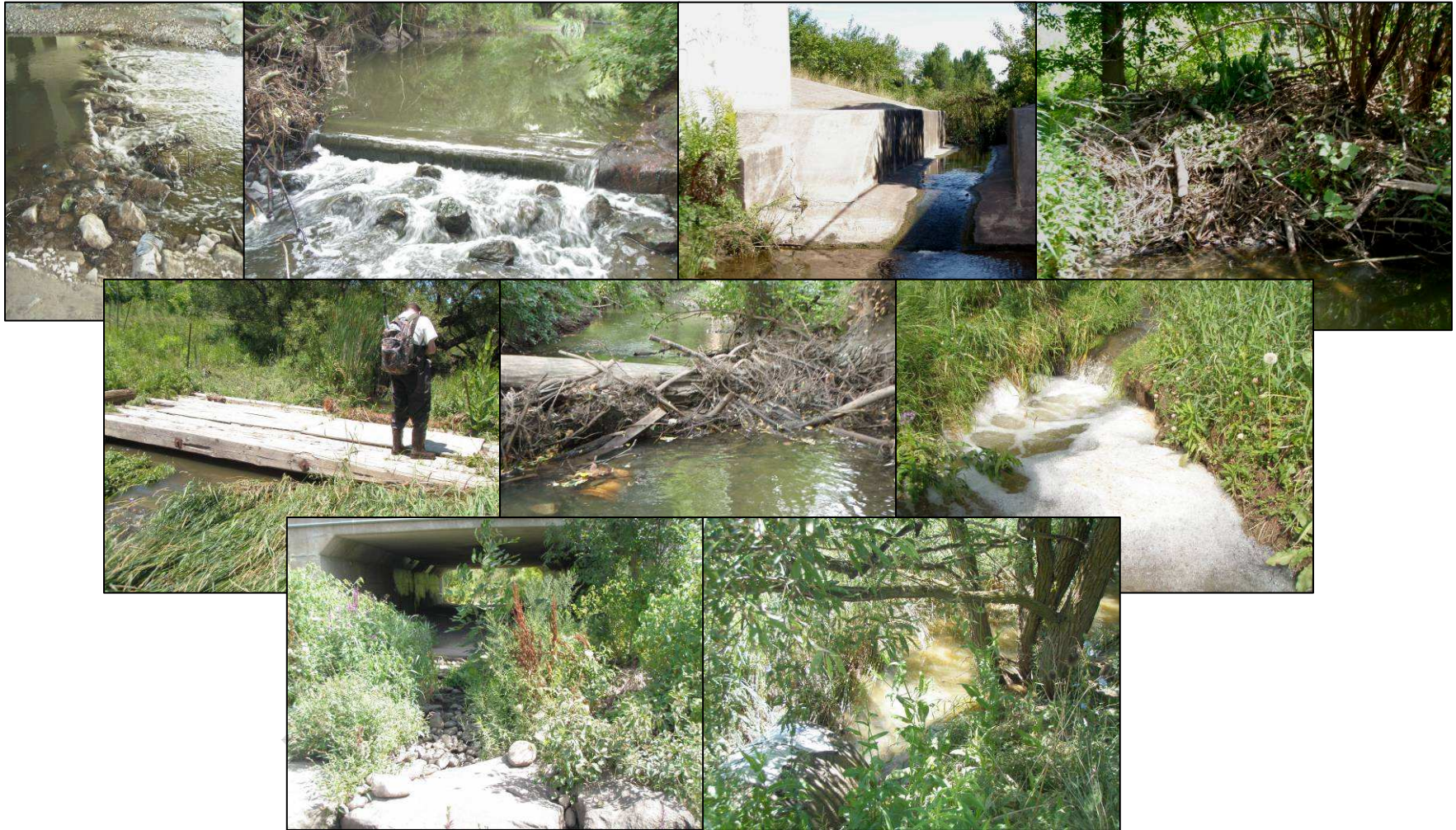
Figure 5.8 Examples of existing fish barriers in Fletcher's Creek
