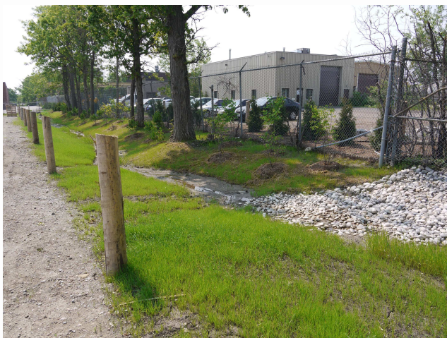
Swale enhancement on the west side of the property
