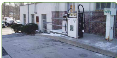
Stormwater runoff from uncovered fueling areas at private fleet management facilities flows directly to nearby storm drain inlets.
