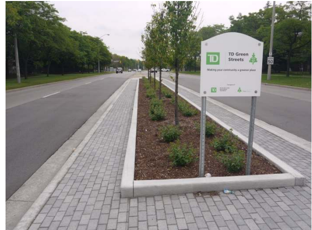
Silva cells help to green Central Parkway in Mississauga, Ontario.
