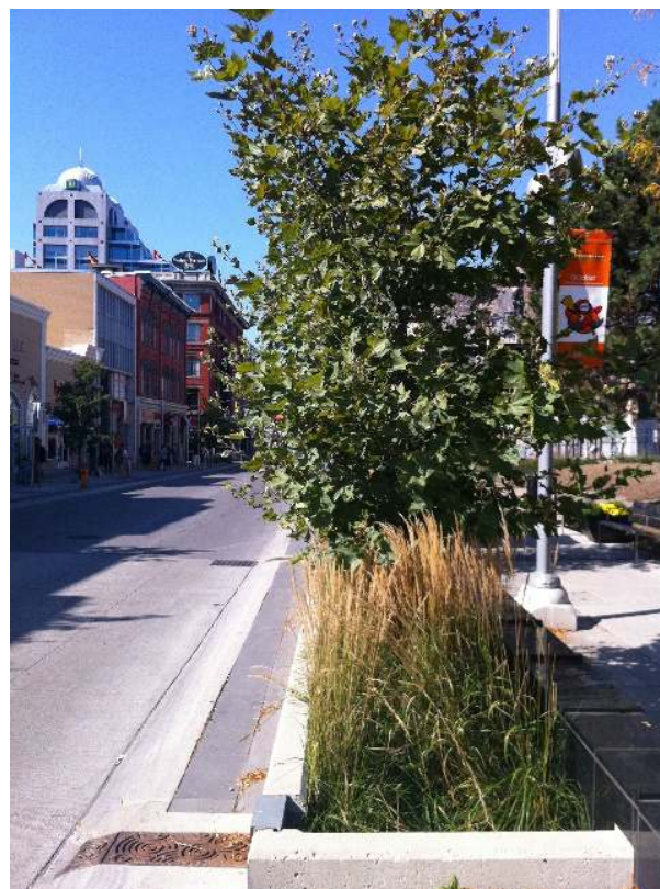
Bioretention planters on King Street in Kitchener.
