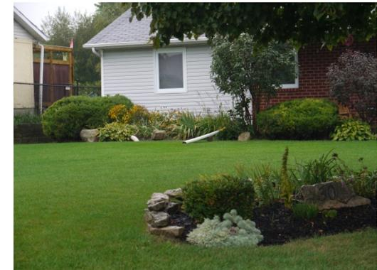
**Figure 6: Roof drainage from this property is directed to a lawn area. The long overland flow path across this relatively flat grassed surface allows for infiltration to occur. (Source: CVC)**
