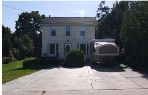
**Figure 5: The drainage pattern on this lot is split. Notice that a significant slope is present on the left side of the home. It would be difficult to direct rear and side yard drainage to the front of the property. (Source: CVC).**
