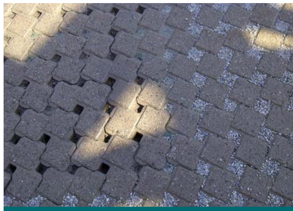
Figure 10.3.3: In this photo the aggregate has been removed from permeable interlocking concrete pavers. This will need to be replenished immediately to avoid clogging of the joints. (Source: Aquafor Beech)
