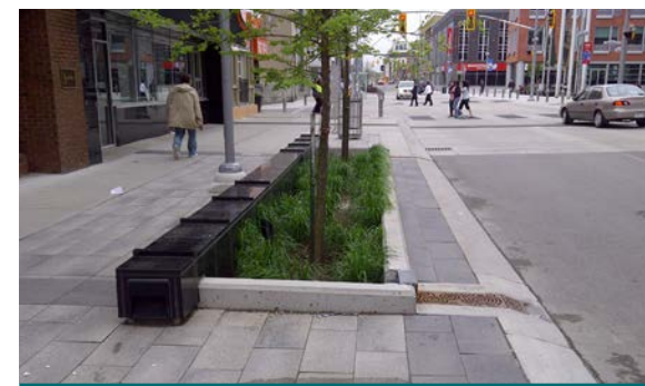
Figure 2.1.1: Bioretention planters can incorporate multiple features. The bioretention planters on King Street in Kitchener provide growing media for street trees, seating for pedestrians, and street lighting (accent lighting within the planters). (Source: Aquafor Beech)
