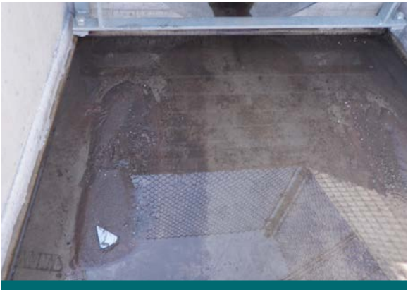
Figure 10.2.4: Along with measuring sediment depth in a proprietary stormwater treatment device, check the outlet structure if accessible. If the OGS is functioning as intended, sedimentation should not be occurring. (Source: Aquafor Beech)
