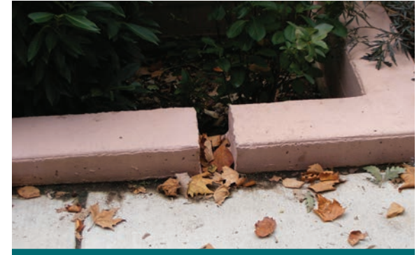
Figure 6.4.6: Notched curb cuts prevent larger debris from accumulating in bioretention planters. A greater number of curb cuts may be required to allow for design flow conveyance. (Source: Aquafor Beech)
