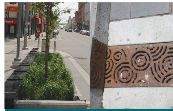
Figure 4.3.31: City of Kitchener incorporated bioretention planters into their main commercial street, King St. The design incorporates seating and trench drains with decorative grating to take runoff from the street. (Source: CVC)
