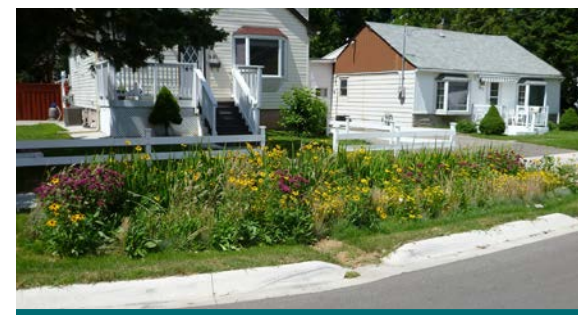
Figure 2.1.7: Boulevard bioretention units are ideally suited for road reconstruction projects upgrading residential streets with a rural cross section to an urban cross-section. This photo shows a home in the Lakeview neighbourhood in Mississauga with a planted boulevard bioretention unit. (Source: CVC)
