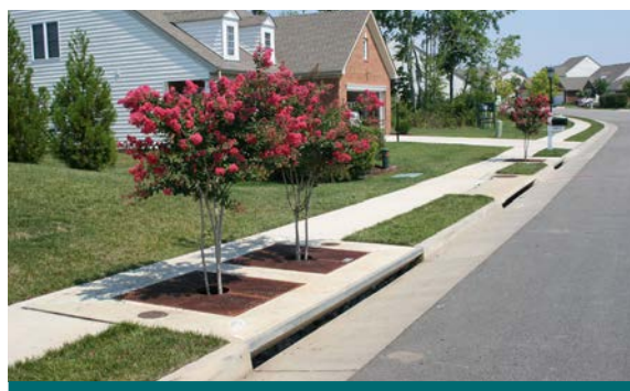
Figure 2.4.1: A Filterra Bioretention System (the flowering plantings and buried precast unit pictured above) is one type of precast tree planter.(Source: Filterra Bioretention Systems)
