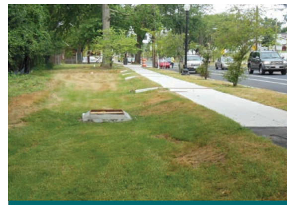
Figure 4.3.20: Grassed bioretention treating road runoff in a wide boulevard space. The grassed bioretention can blend with a corporate property lawn and will be easy for property maintenance staff to maintain with little to no training. (Source: CVC )
