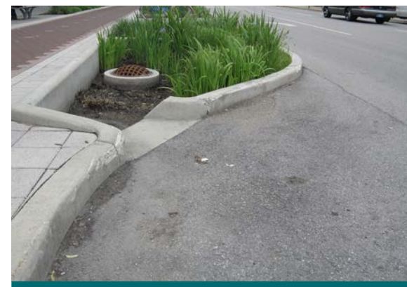
Figure 2.1.5: Curb extensions can be built to accommodate existing locations of stormwater management infrastructure, such as catch basins. (Source: CVC)
