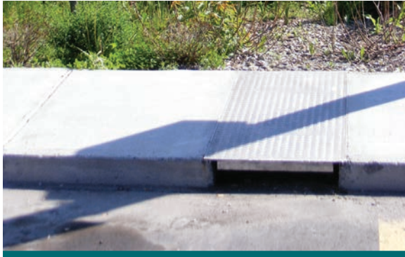
Figure 6.4.2: Ensure that grates are corrosion resistant and have anti-slip measures. (Source: Aquafor Beech)
