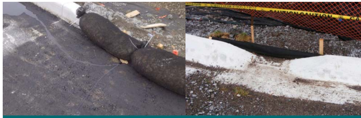
Figure 11: Sediment logs used for erosion and sedimentation control at curb cut locations during construction. (Source: Aquafor Beech)
