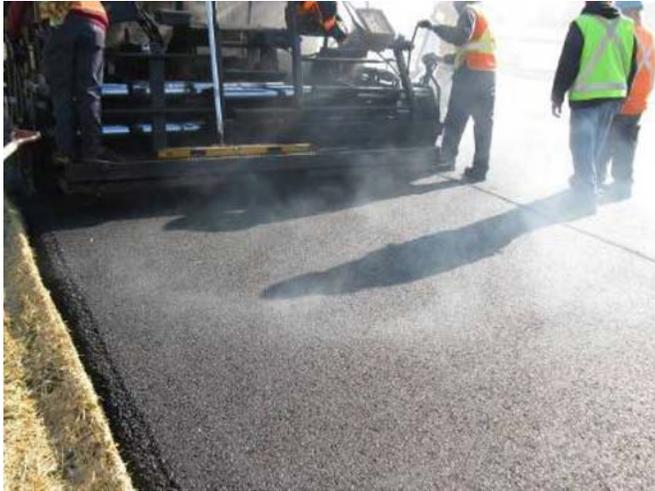
Installation of rubber modified asphalt test strip
