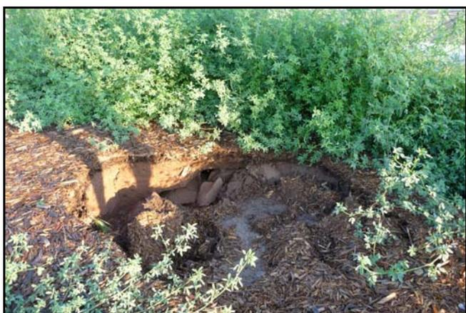
Image of a surface depression that formed within the bioretention cell shortly after construction
