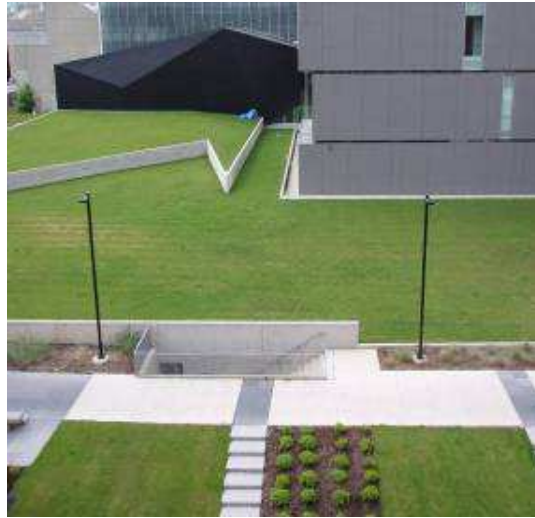
University of Toronto - Mississauga Campus - green roof (photo credit: CVC)
