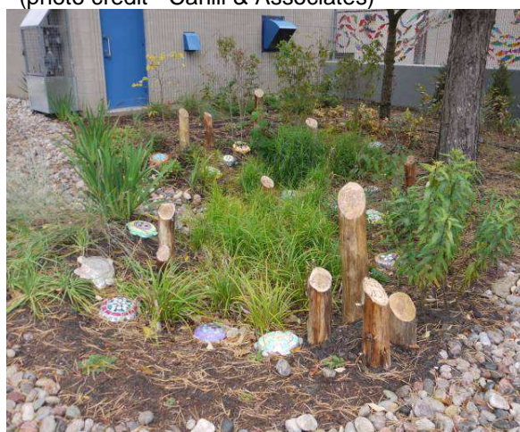
Green Glade Public School in City of Mississauga - bioretention cell taking parking lot runoff and roof runoff (photo credit: CVC)
