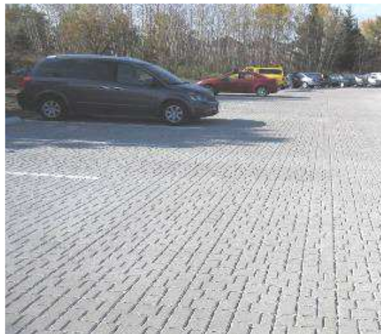
CVC Main Office in the City of Mississauga - interlocking concrete permeable paver lot (photo credit – CVC)
