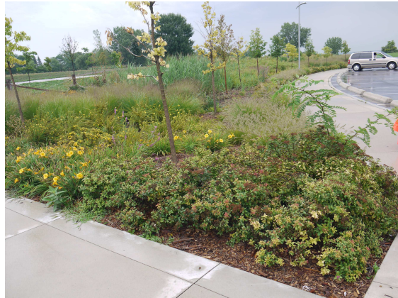
Lakeside Park in City of Mississauga - dry swale or bioretention swale taking runoff from parking lot. Photo credit: Seattle Public Utilities
