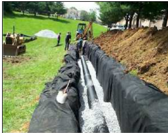
Rear lot infiltration trench under construction. (photo credit - Cahill & Associates)
