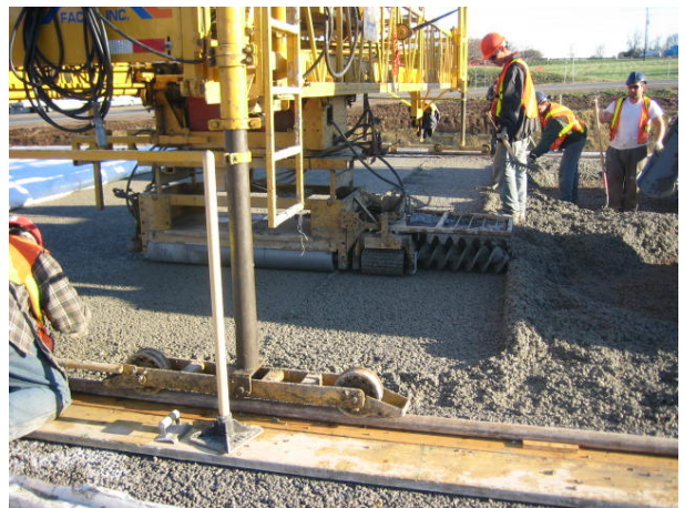
Bid-well deck paver tested for pervious concrete placement
