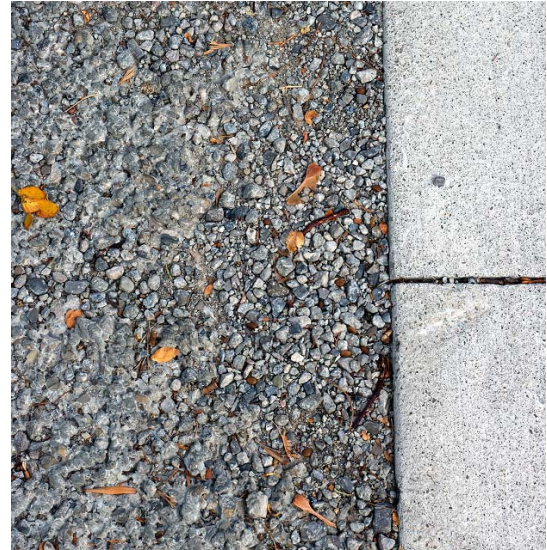
Example of pervious concrete raveling (note the loose aggregate near the curb)
