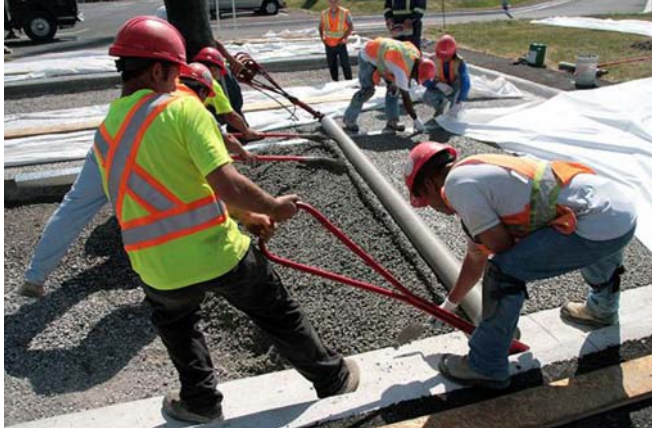
Installation of pervious concrete by hydraulic roller screed
