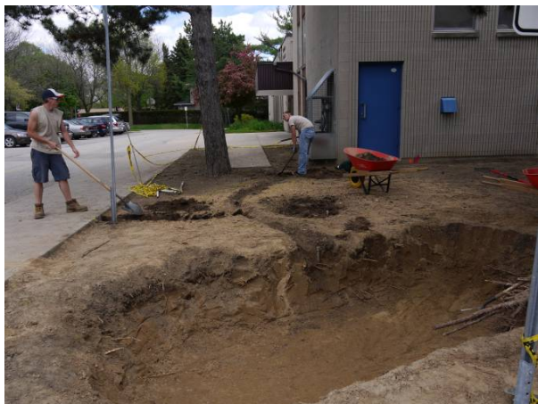
Excavation Work Being Conducted at Rain Garden
