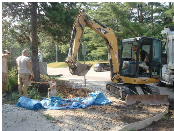
Removal of the soil media with mini-excavator
