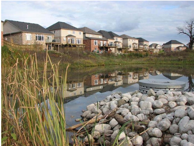
Picture of stormwater management pond used to pre-treat stormwater prior to infiltration via kettle depressions
