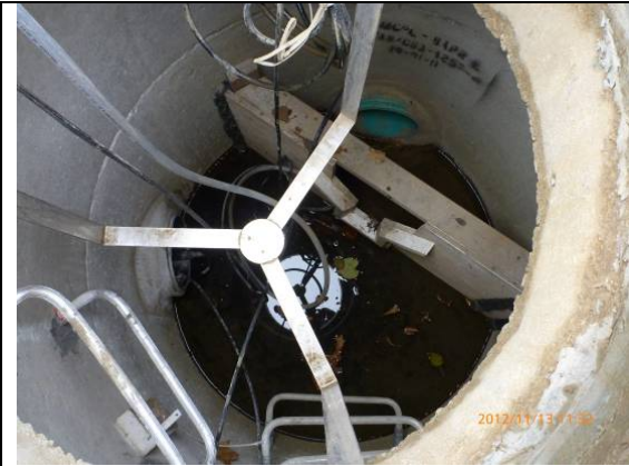
November 13, 2012 – Monitoring manhole
