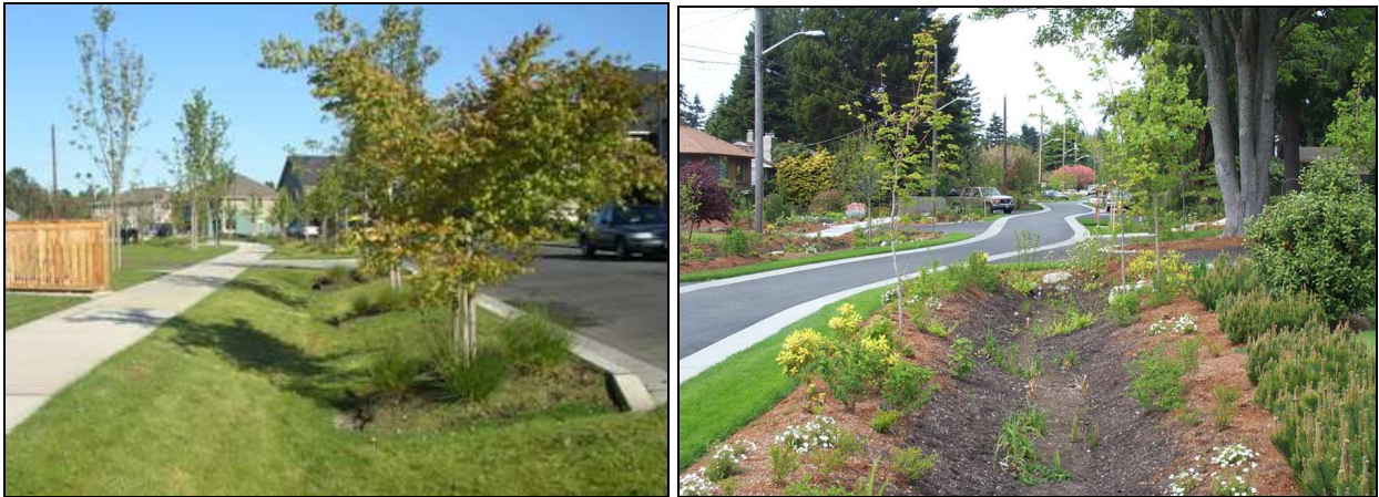
Figure 4.9.1 Dry swales can be vegetated with turf grass or more elaborate vegetation
