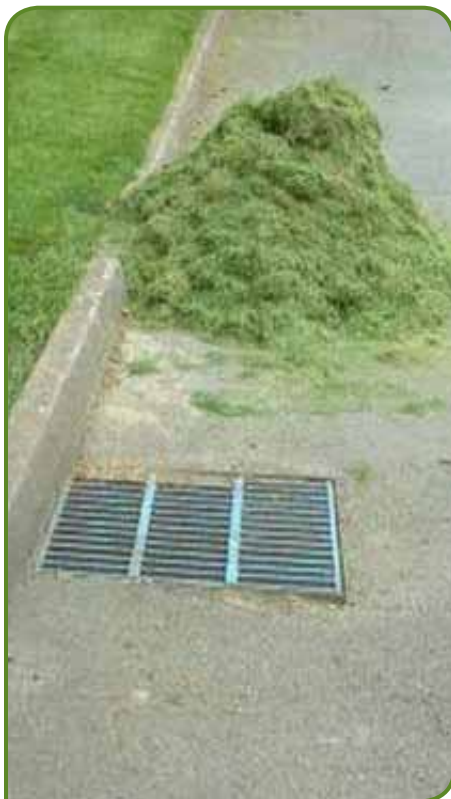
Dumped grass clippings may clog the storm drain inlet.
