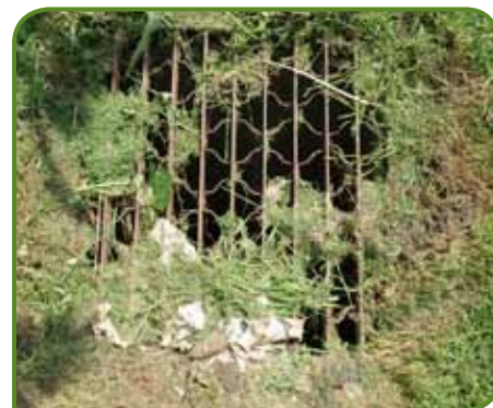
Dumped grass clippings may clog the storm drain inlet.
